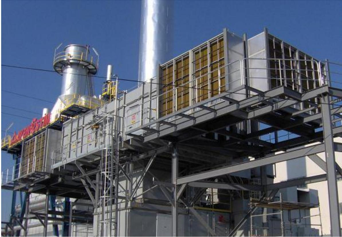
**Picture.2- Sample Application of a Combustion Turbine Inlet Air Cooling Unit**
