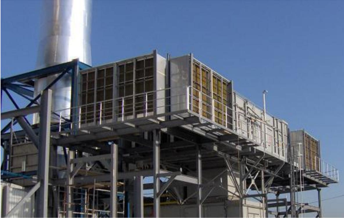
Picture.3- Sample Application of a Combustion Turbine Inlet Air Cooling Unit
