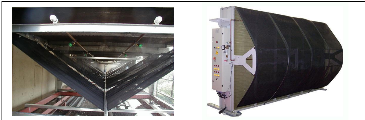
Figure 1.A, 1.B. Vertical and Flatbed Mesh and Spray System Air Cooled Condensers [3], [1]
